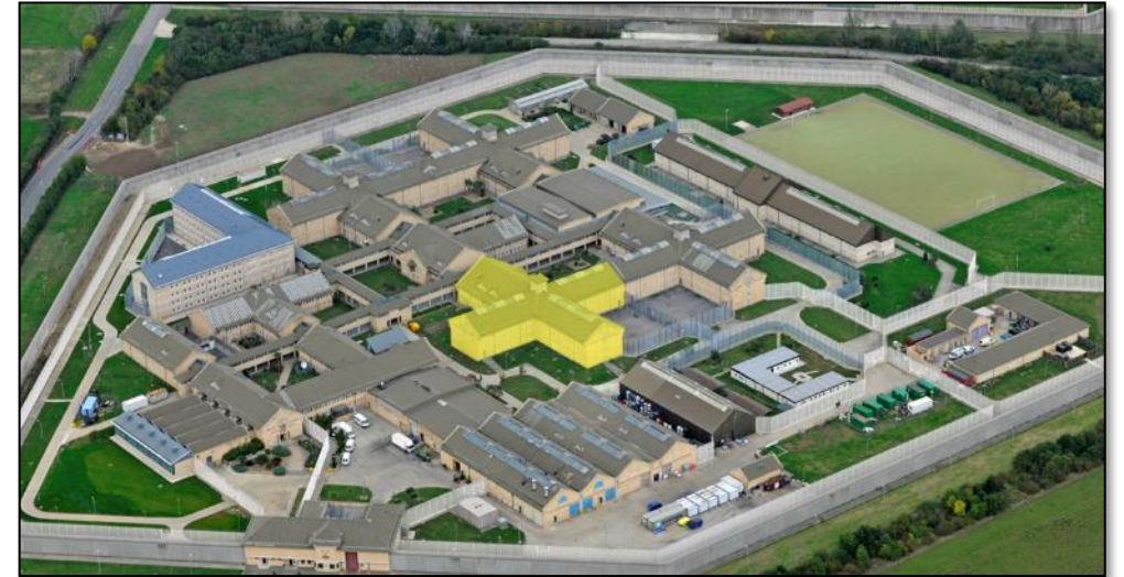
HMP Elmley – Houseblock 2 – Phase 1
